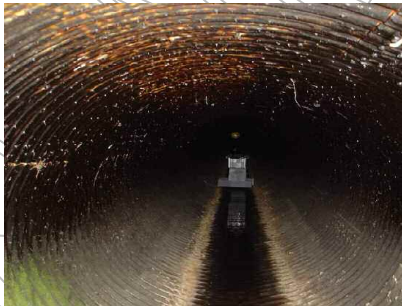
Image 5.3 Automated bat detector placed within a culvert to record bat activity. Ensure that equipment will not obstruct watercourse culverts. Lesser horseshoe bats are currently using this to fly underneath a dual carriageway on embankment.
