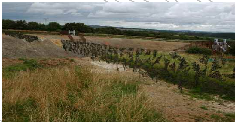
Image 8.17 Temporary structure using wire and camouflage netting constructed over a cutting during construction of a new dual carriageway to reconnect an important bat flyway.
