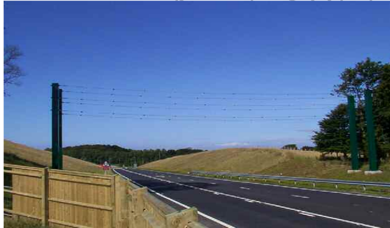
Image 8.14 Wire structure. Success is only likely to be possible if they are erected in conjunction with existing roadside trees. This example could be improved by bridging the gap to adjacent vegetation.
